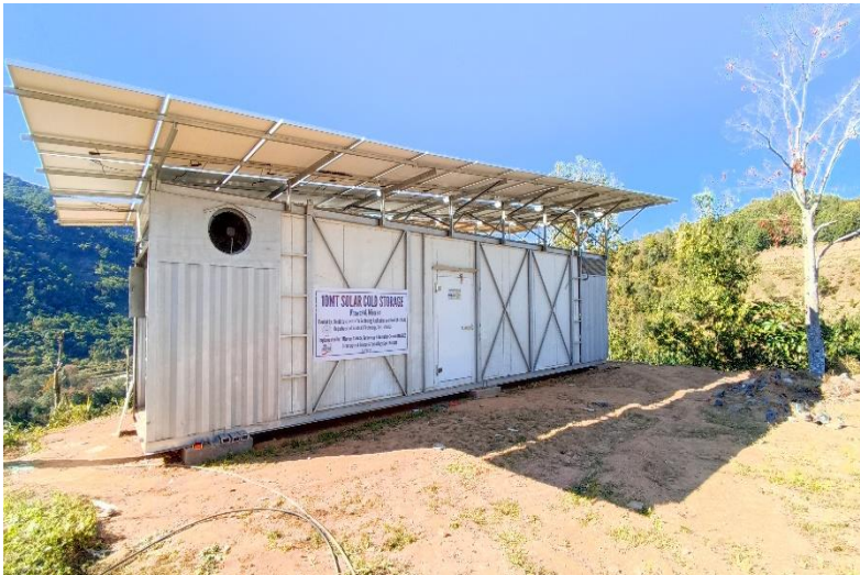
Solar Cold Storage at KVK, Khawzawl
