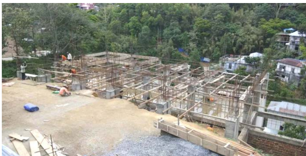
The Centre building is now under construction
