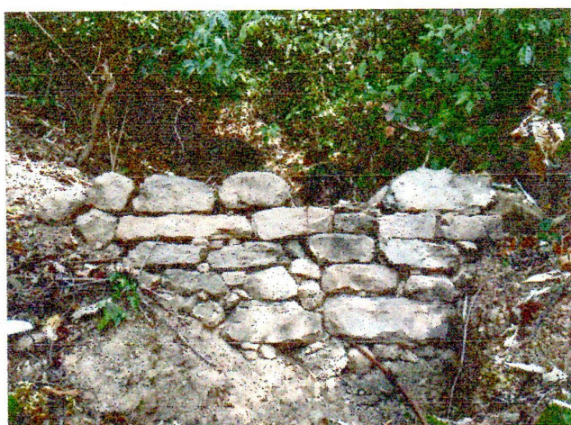
Loose boulder Checkdam
