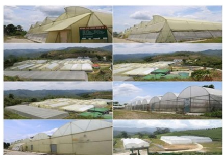
Fig. 5a. ). Infrastructure for Protected Cultivation at Lunglei District
