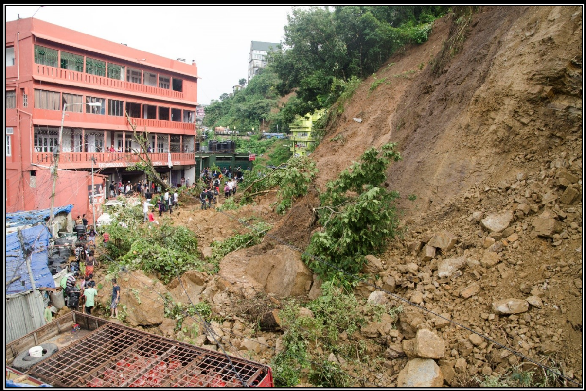
Landslide at Bawngkawn, Aizawl cutting off vehicular movements
