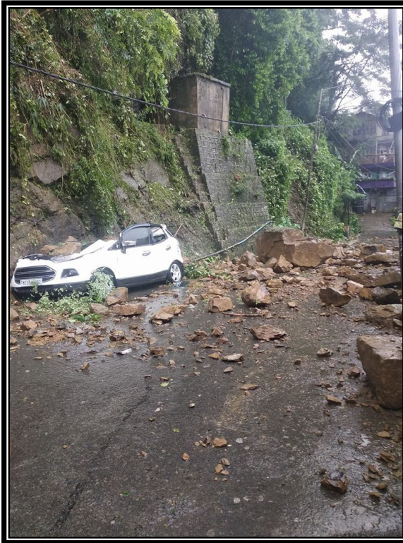
Rockslide at Chanmary West, Aizawl
