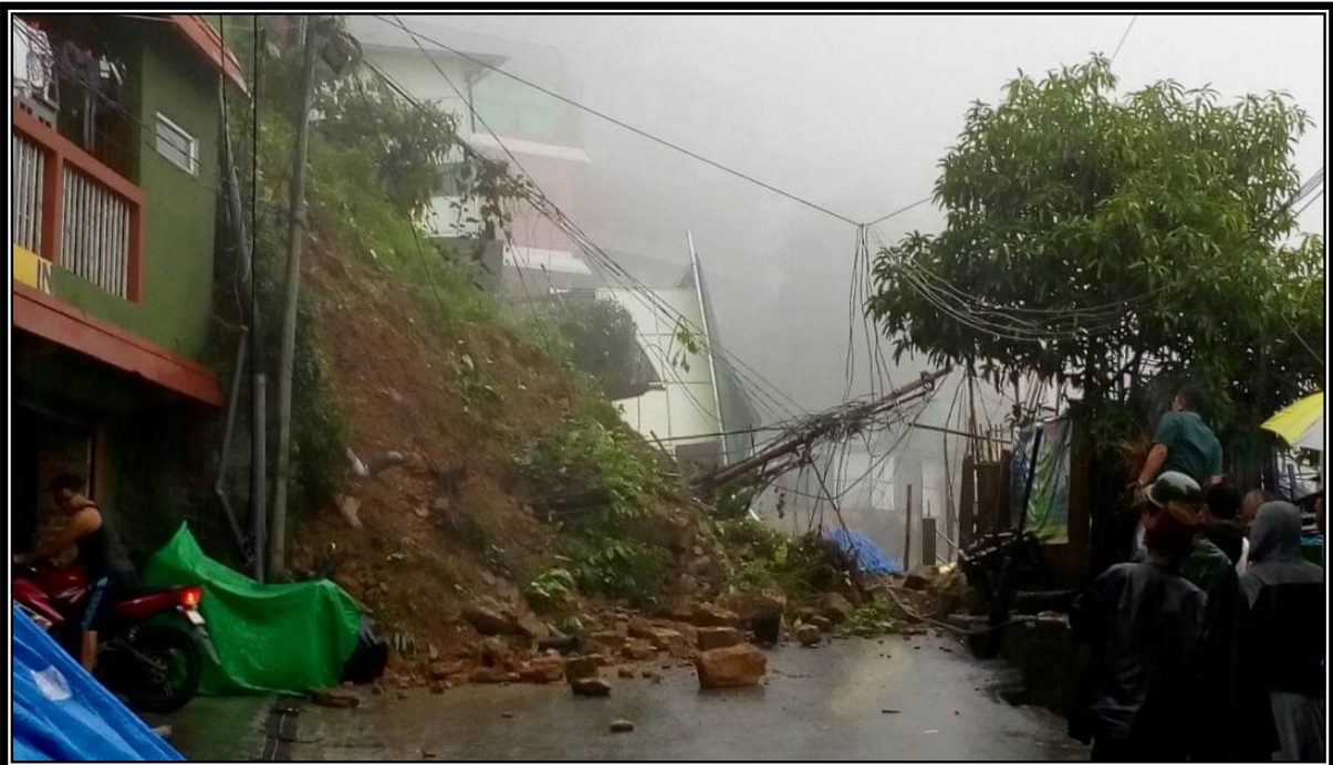
Landslide at Tuithiang Veng, Aizawl
