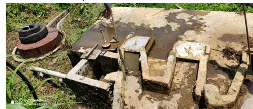
Installation of Bio Gas to reduce from emission of gas (methane)
