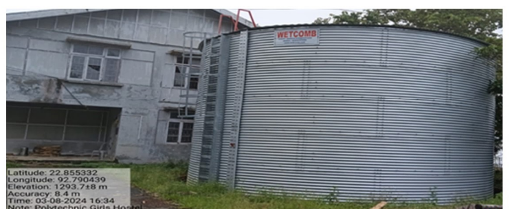
Rooftop Rainwater Harvesting at Lunglei
